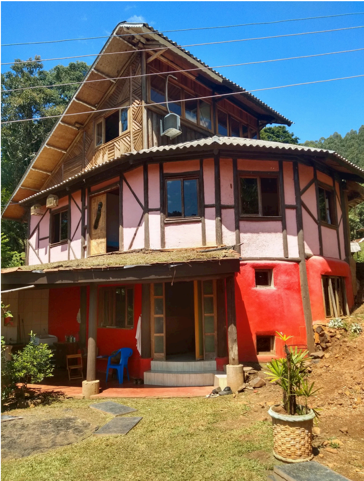
Figure 9. Residence built with wooden structure, wattle and daub and bagged earth walls, and a green roof. Source: Architect - Cecilia Prompt. Photo by Cecilia Prompt.
