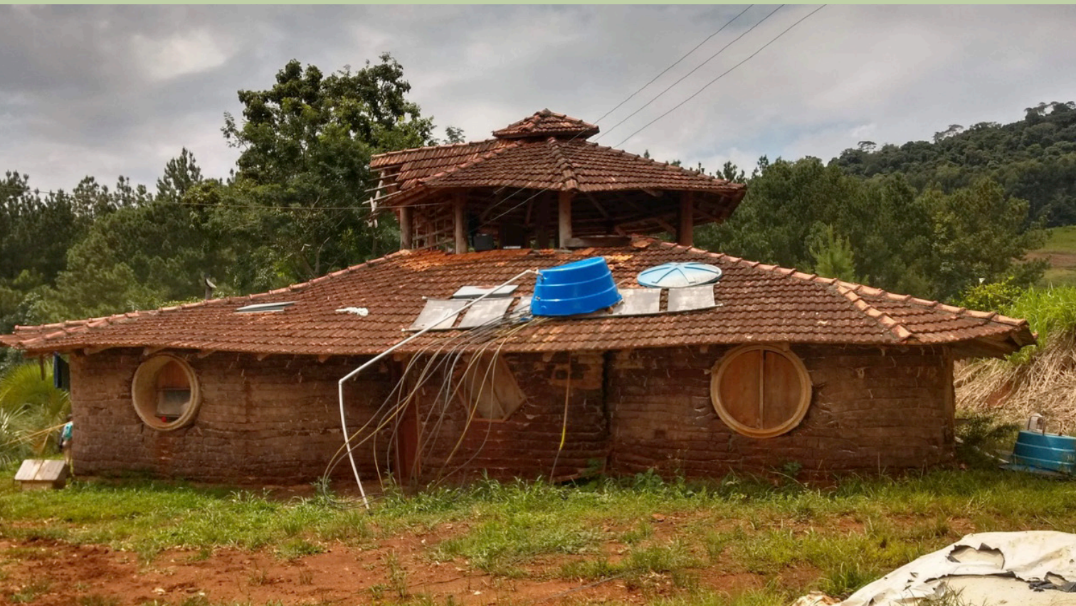
Figura 0. Residence built with bagged earth and wattle and daub walls. Source: Architect - César Costa. Photo by Cecília Prompt.
