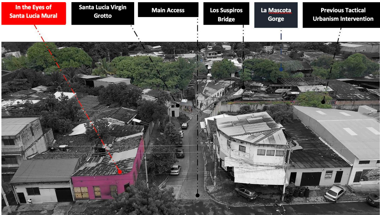
Figure 5. Significant elements of the Santa Lucia Community. Source: Preparation by the authors.
