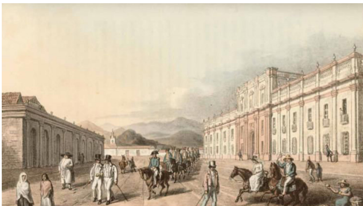
Figure 4 Ideal reconstruction of the facade integrating the crest of Andía and Varela, and the insignia and shields removed in 1822.
