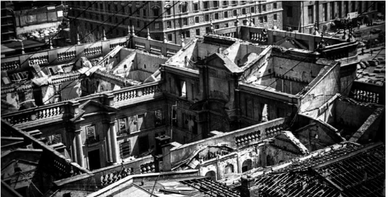
Figure 12 Overhead view of Palacio de la Moneda after the bombing, by DA MOP (1973). Source: DARM MOP (2014).
