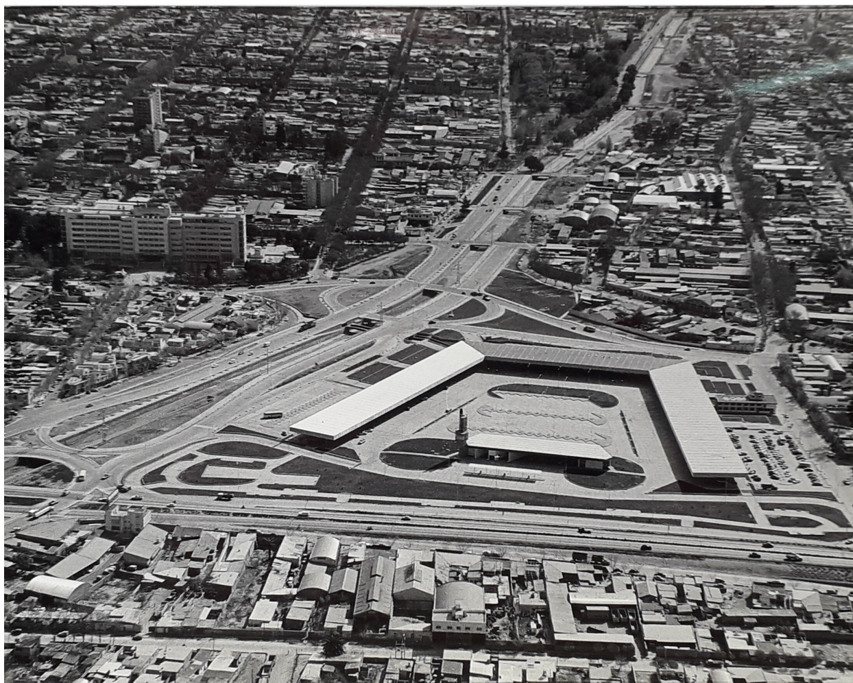
Figure 1. Panoramic photo of the Terminal. Source: Personal archives of architect Gilberto Olguín (1972).
