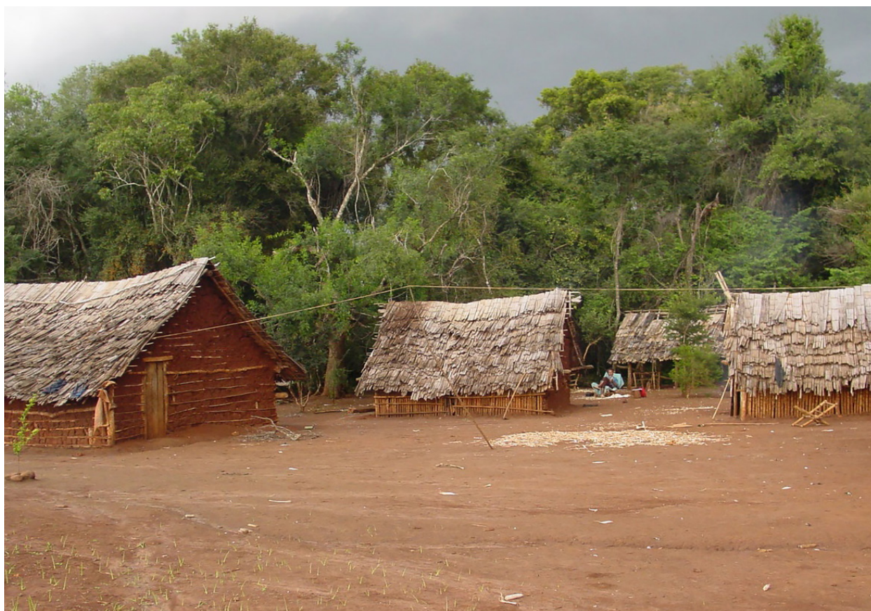
Figure 1. Set of homes and opy , Tekoá Koenju . The buildings have the colors of the Earth used as enclosures for the walls. The roofs and structures comprise local plant species with symbolic meaning. Source: Zanin, 2006.
