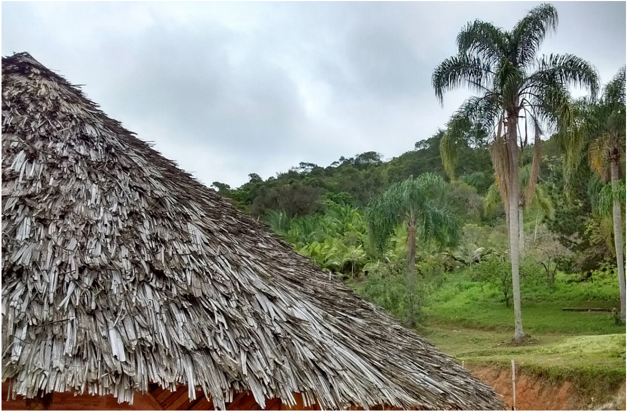
Figure 3. Opy covered with taquara and set of pindó in the surroundings, Tekoá Yynn Morotchi Wherá. Source: Zanin, 2021.
