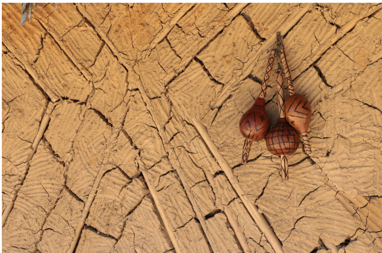
Figure 4. Detail of the Tekoá V'a opy wall. Detail of the Tekoá V'a opy wall, on light-colored raw land, due to its proximity to the coast. The marks left by the fingers that smoothed the wall can be seen, a trait of the traditional Guarani construction process. Source: Zanin, 2021.
