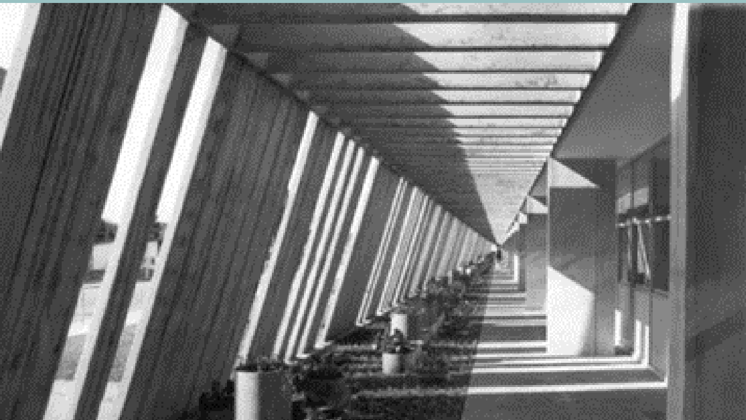
Figura 0. Second Army HQ internal facade photo (1969) Source: Paulo Bastos Archive.
