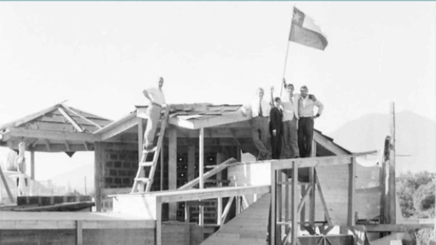
Figure 0. José Vial during the construction of the house in Jean Mermoz, 1960. Source: Archive Historical José Vial Armstrong.
