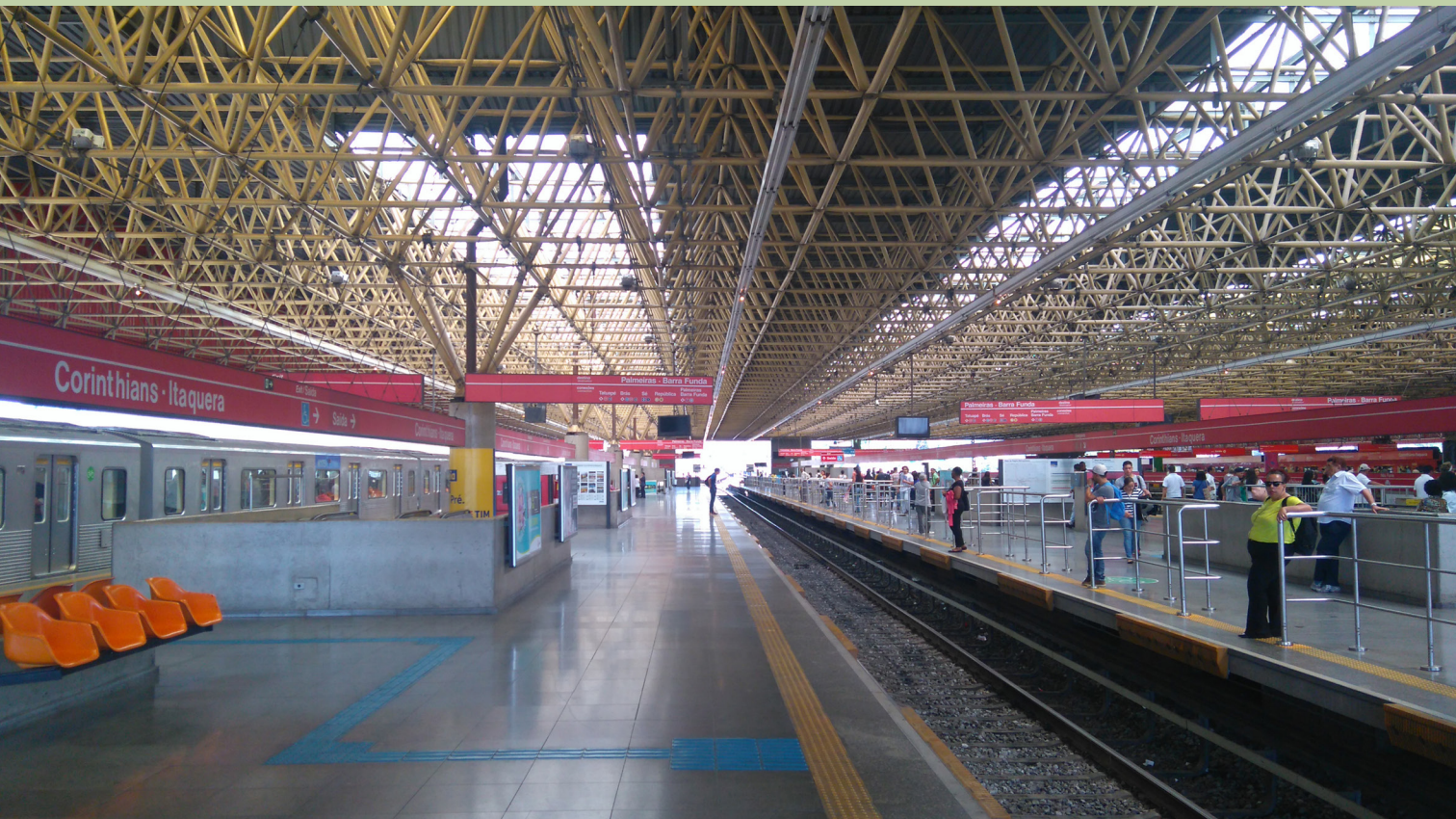
Figure 0. Views of the subway platform and roof from inside the station. Source: Author's photo in 2017.
