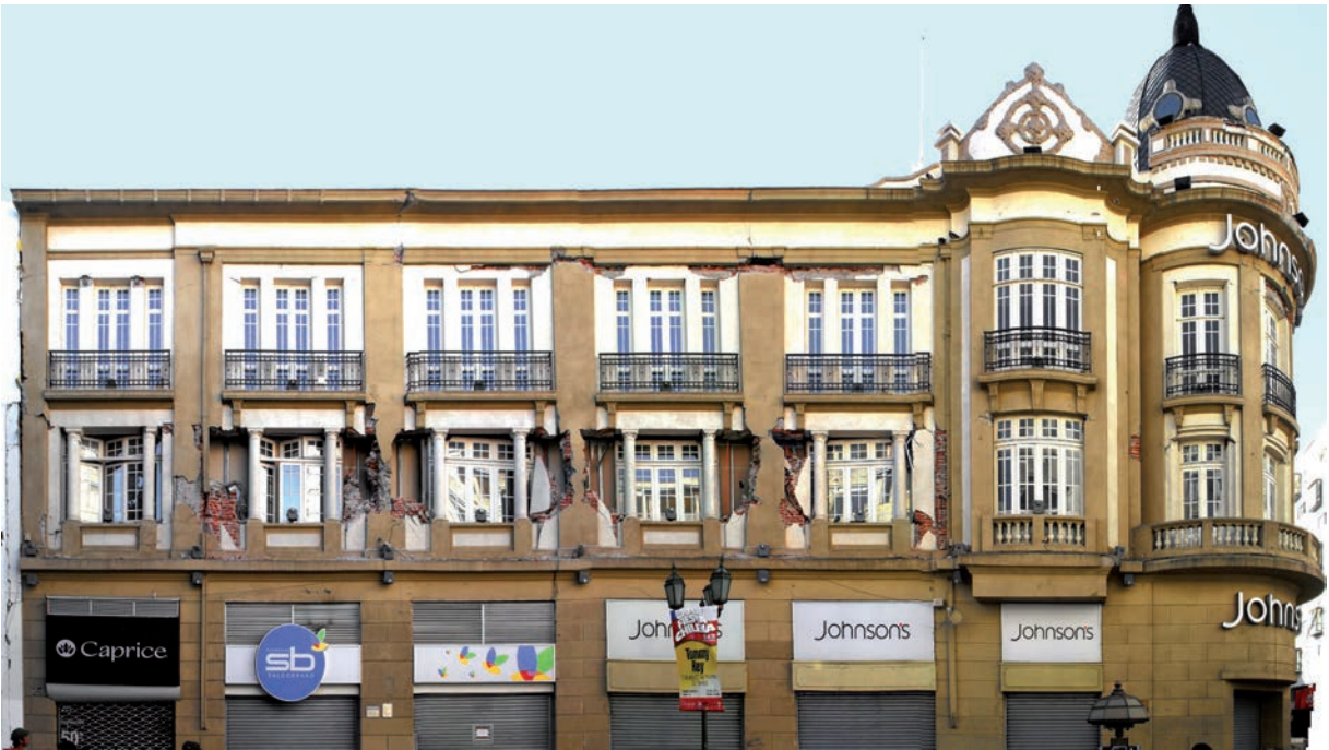
Figura 13a A 18 días del terremoto. Esquina calles Barros Arana y Colo Colo. Antiguo "Palacio Hirmas", edificación de fachada-continua estructurada a base de ladrillo que alberga recintos comerciales. / Eighteen days after the earthquake. Corner of Barros Arana and Colo-Colo. Former 'Hirmas Palace', brick street front building that used to house commercial dependencies.
