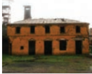
[02] EDIFICIO LAMPARERÍA THE LAMP BUILDING
