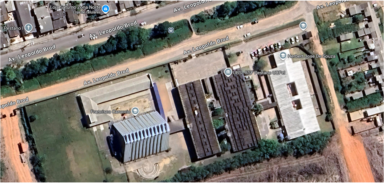
Figure 5. Aerial view of the building that would be the CAIC of Pelotas. Source: GeoPelotas, 2022.
