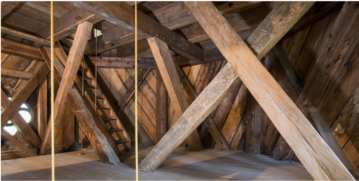
Figure 14. Bell tower structure with sighting of joint recess and use of dowels. Source: Oficina Plan Arquitectos.
