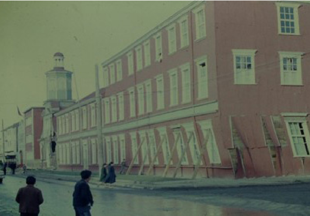
Figure 5. Image of the San Francisco Javier School with the damage from the 1960 earthquake. Source: Fabregas Zelada (2022).
