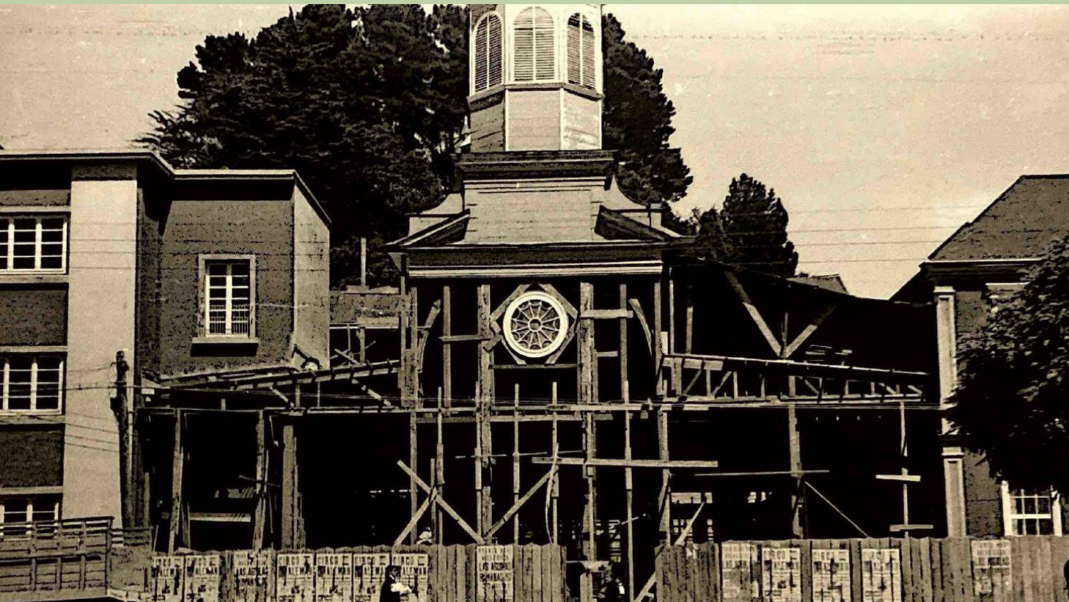
Figure 0. Church facade under repair, 1962. Source: Castro Fones & Brauning Salazar (2022).
