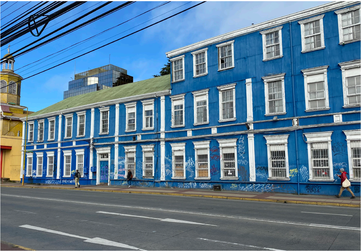
Figure 3. Image of the facade of the San Francisco Javier School. Source: Obando Aedo (2024).
