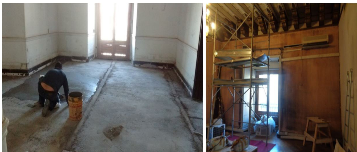
Figure 15 Conservation works South Wing (2016 – 2018). Source: DARM MOP (2016).
