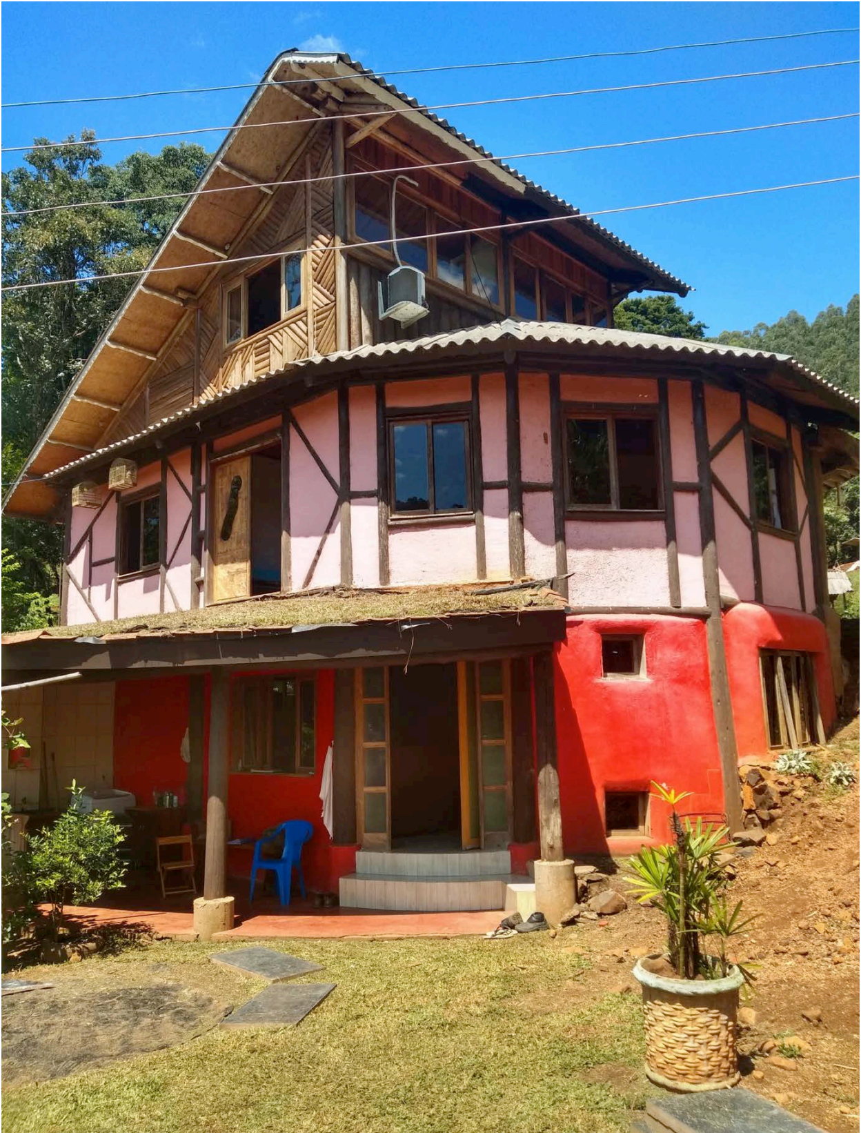
Figure 9. Residence built with wooden structure, wattle and daub and bagged earth walls, and a green roof. Source: Architect - Cecilia Prompt. Photo by Cecilia Prompt.
