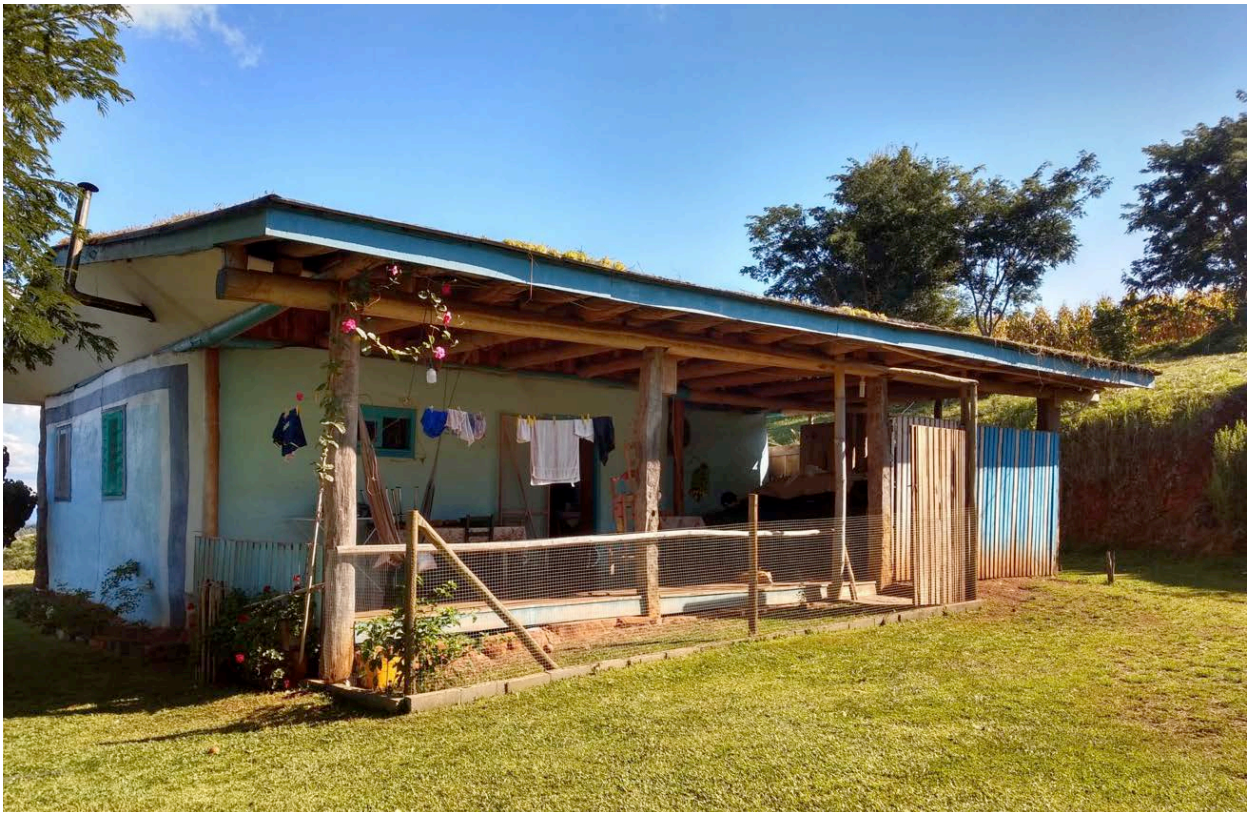
Figure 4. Residence built with bagged earth and a green roof. Source: Architect - Silvio Santi. Photo: Cecilia Prompt.
