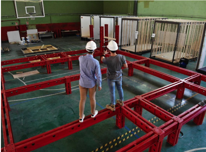
Figure 11. Beginning the prototype's construction. Source: Preparation by the authors.
