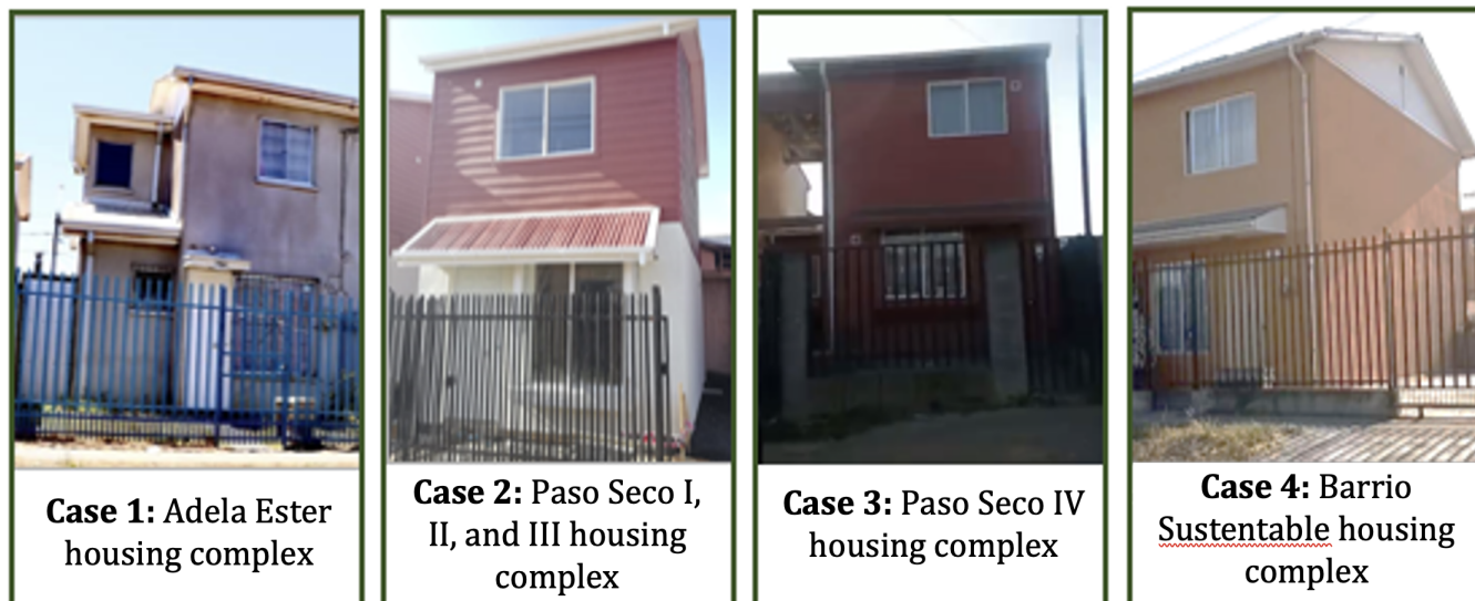
Figure 2. Images of the main facades of the cases chosen as a sample. Source: Preparation by the authors.
