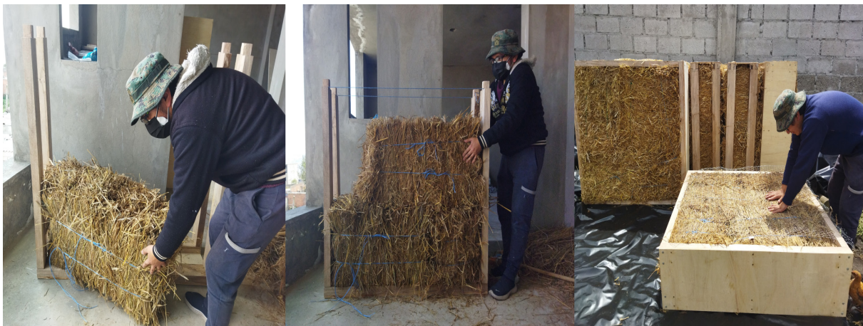
Figure 10. Construction of panels Source: Preparation by the authors.
