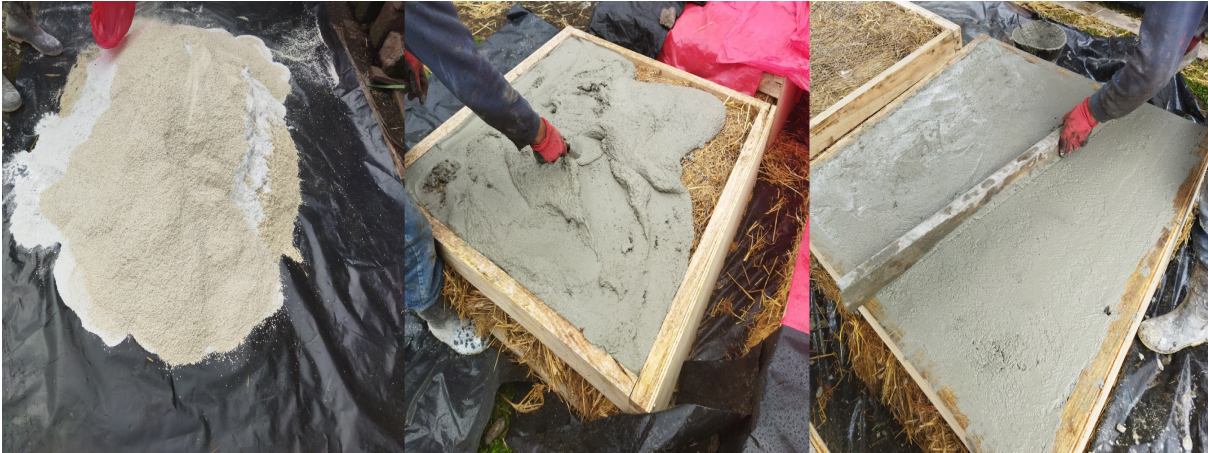
Figure 11. Application on mortar panels made with 5050AM2 mixture. Source: Preparation by the authors.
