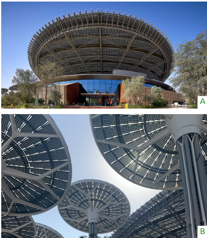
Figure 11. Sustainability pavilion exterior canopy made of steel and (B) photovoltaic trees that are nature-based in form and function. Source: Fairs, 2021; Prisco, 2021.
