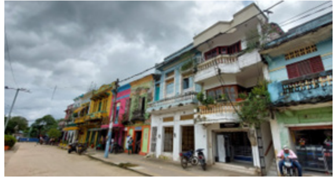
Figure 11. Urban masonry houses, Sucre. Source: Preparation by the authors.
