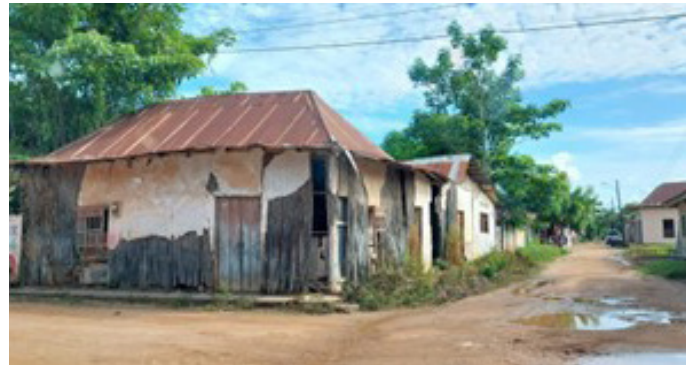
Figure 13. Traditional urban house using American oil palm, Santiago Apostol. Source: Preparation by the authors.
