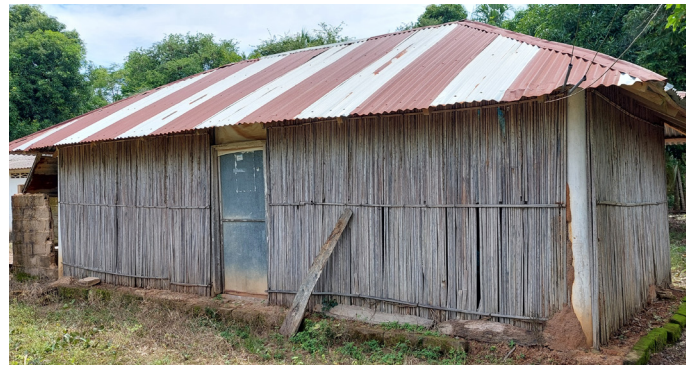
Figure 15. Traditional house in the marsh using American oil palm, San Marcos. Source: Preparation by the authors.
