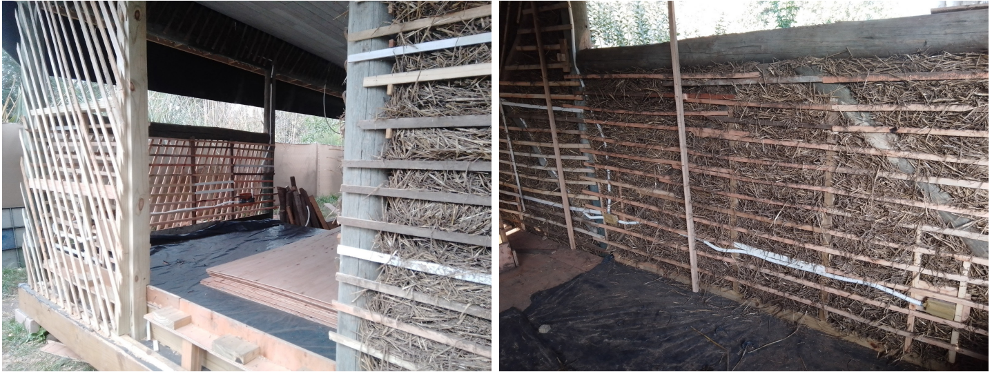
Figure 3: Housing construction process - Escobar. Source: Preparation by the authors.
