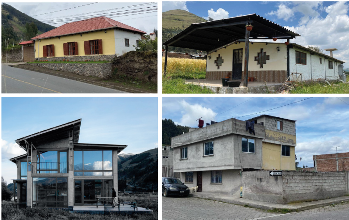
Figure 2. Selected case studies: (a) TRA-01 traditional brick dwelling; (b) TRA-02 straw bale dwelling; (c) CON-01 brick dwelling; (d) CON-02 concrete block dwelling. Source: Preparation by the Authors.
