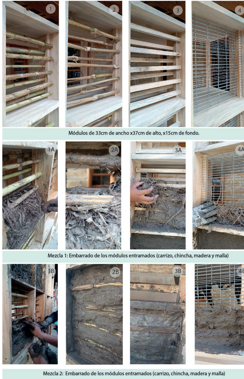
Figure 2. (a) Floor plan and elevation of the truss sampler. (b) Preparation of the dosed mixture. (3) Application of the mixture in the reeds, chinchá, wood, and mesh structures. Source: Preparation by the Authors.
