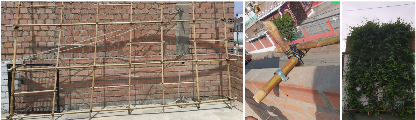
Figure 7. Assembly of the structural system of the bambucillo and installation on the wall. Source: Prepared by the authors.
