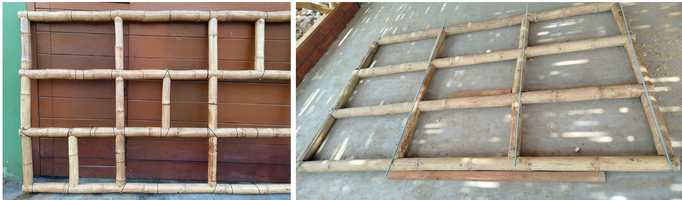
Figure 6. Assembly of the bamboo structural system. Source: Prepared by the authors.
