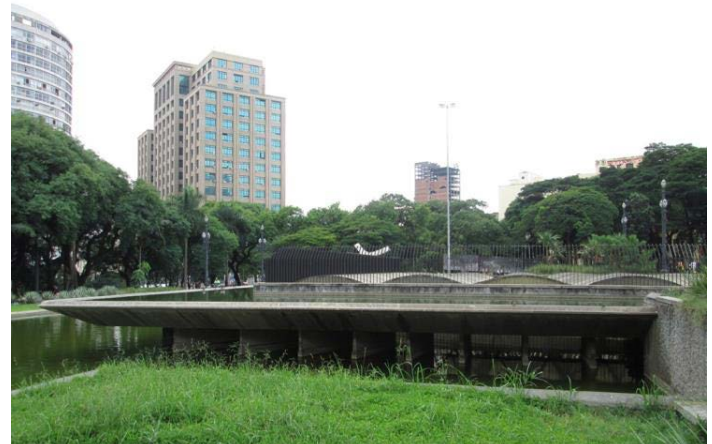
Figura 7. Link between Praça da Sé and Sé Station. Source: Author photo
