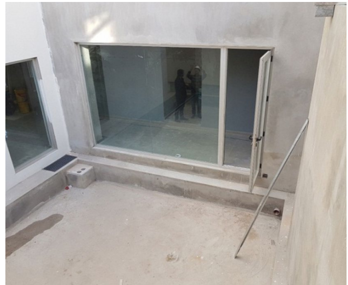
Figure 4. Hydraulic control device. Source: Left: Santa Fe Water Resources Secretariat. Figure 5. Reservoir designed in the building, SJ-58 Pilay-Capitel, Irigoyen Freyre 2230, Santa Fe. The ground floor yard is, in itself, the reservoir, and covers its entire surface. Source: Photograph by the authors.
