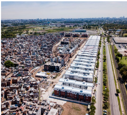
a) Progress of the works, 2019.
