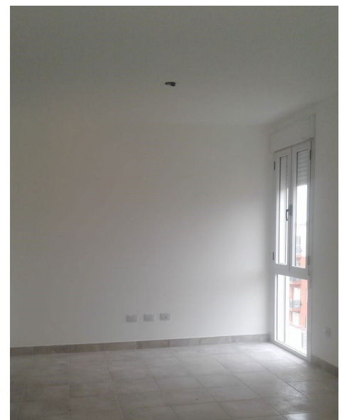
c) Indoor Surface finish and aluminum opening
