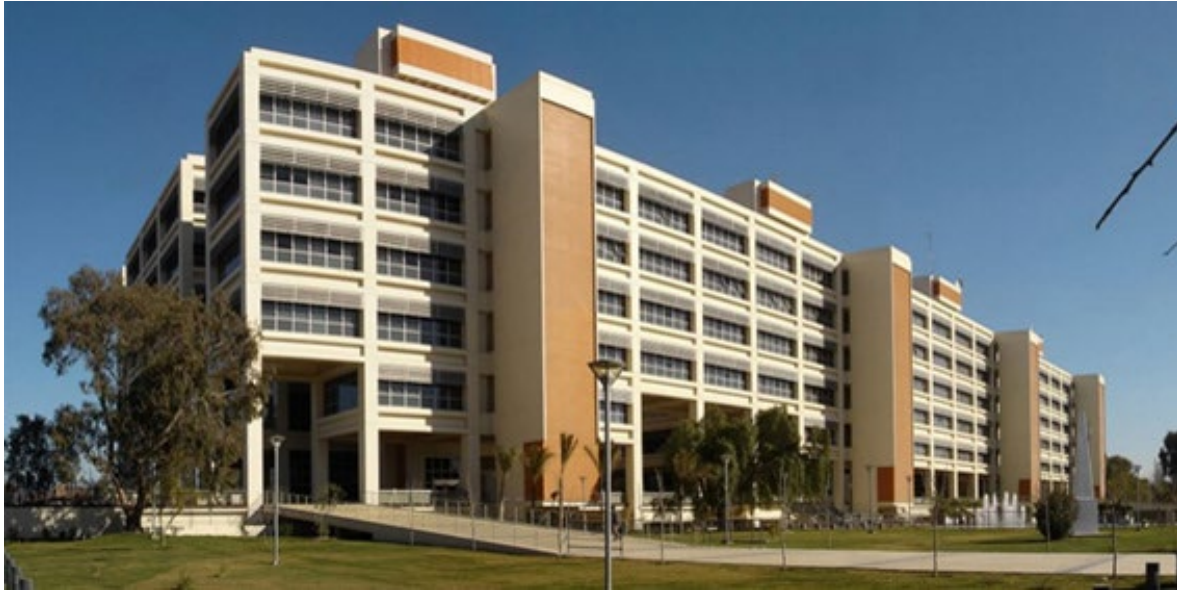
Figure 7. East facade Civic Center Building. Source: Preparation by the Authors. Source: Preparation by the Authors.
