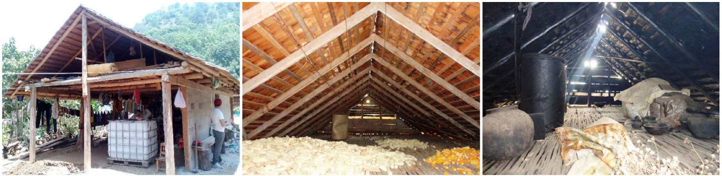
Figure 4. Tapancos in rural areas of Querétaro. Source: Preparation by the authors.
