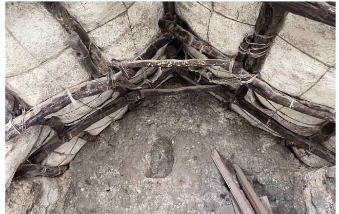
Figure 2. A ceiling of a traditional house in Guallatire, "caruna" or "takta," the material under study is white; photograph from 2022. Source: Preparation by the authors
