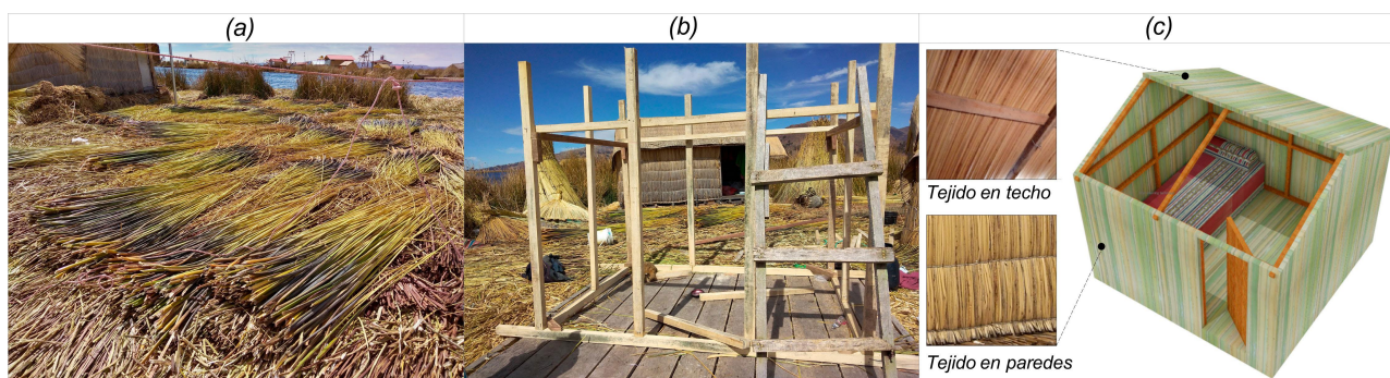
Figure 2. Uro Dwelling - Assembly. Source: Preparation by the authors.
