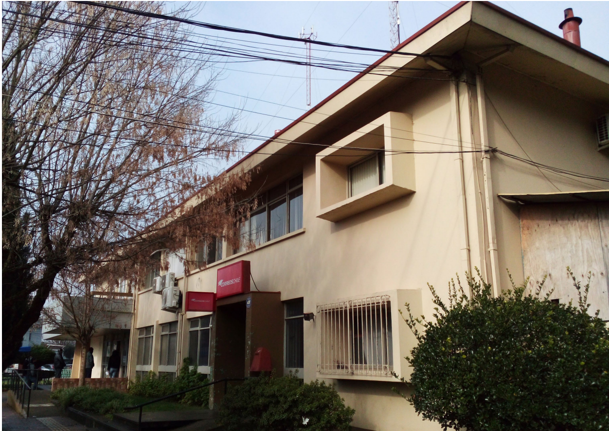
Figure 9. Public Services Building and Municipality of Pitrufoquén. 1974. Source: Gonzalo Cerda Brintrup, personal files, 2023.
