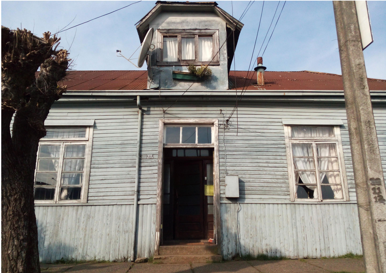
Figure 8. Wooden architecture in Pitrufrquén. Source: Gonzalo Cerda Brintrup, personal files, 2023.
