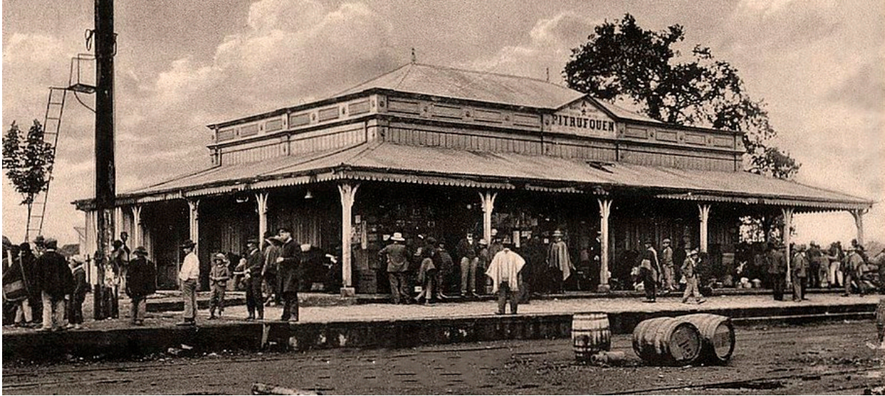
Figure 3. Pitrufoquén railway station, c.1900. Source: Images of Chile from 1900 (n.d.).
