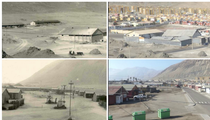
Figure 6. Comparative panoramas between the buildings and original neighborhoods of The Chile Exploration's Company town and the contemporary scene that expresses the urban expansion of Tocopilla, a consequence of the dissipation of the thermoelectric company's territorial control. Source: Author's files, preparation by the author.
